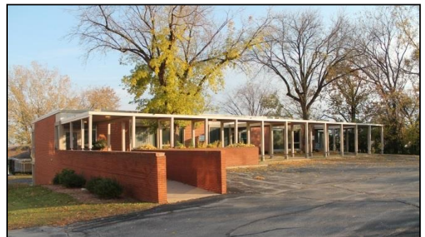
Financial Plaza Building #2, 1961 1825 S. Webster Avenue
