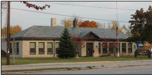
Allouez Water Department, 1947 2143 S. Webster Avenue
