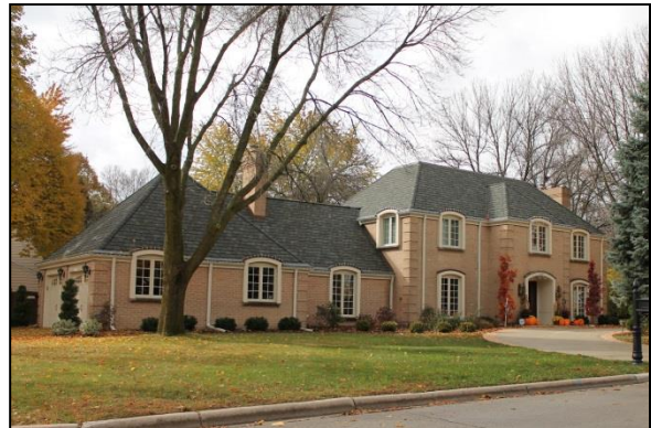
Jack L. Tuttle House, 1976 500 Terraview Drive
