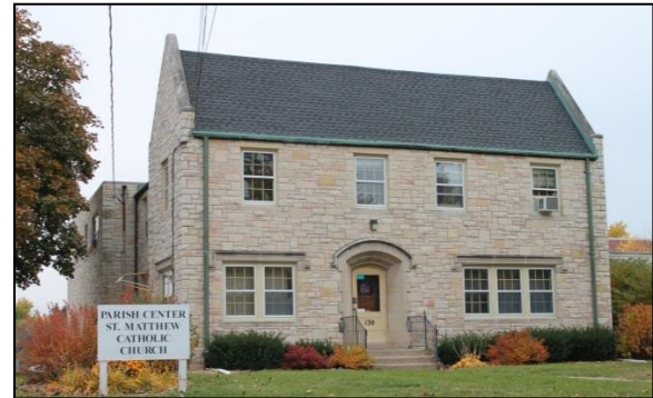
St. Matthew Catholic Church Rectory, 1933 130 St. Matthews Street
