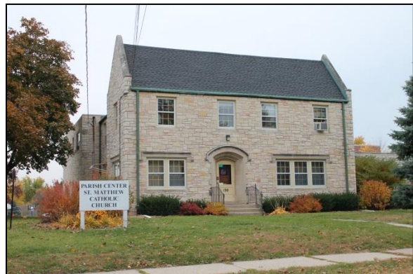
St. Matthew Catholic Church Rectory, 1933 130 St. Matthews Street
