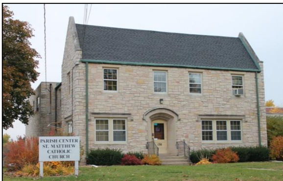
St. Matthew Catholic Church Rectory, 1933 130 St. Matthews Street
