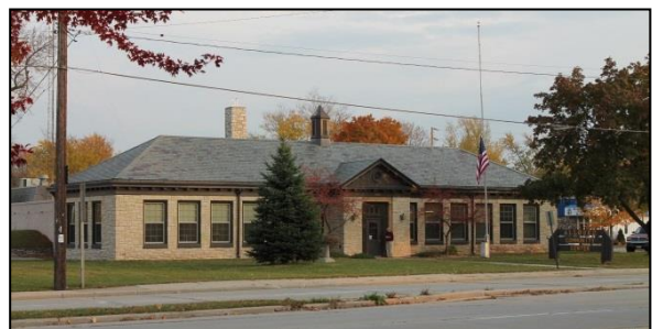
Allouez Water Department, 1947 2143 S. Webster Avenue
