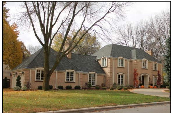
Jack L. Tuttle House, 1976 500 Terraview Drive
