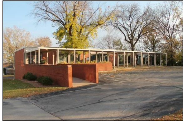
Financial Plaza Building 2, 1961 1825 S. Webster Avenue
