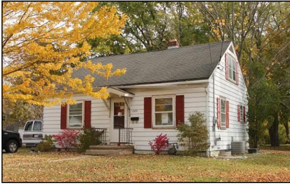
House, 1946 2323 Libal Street
