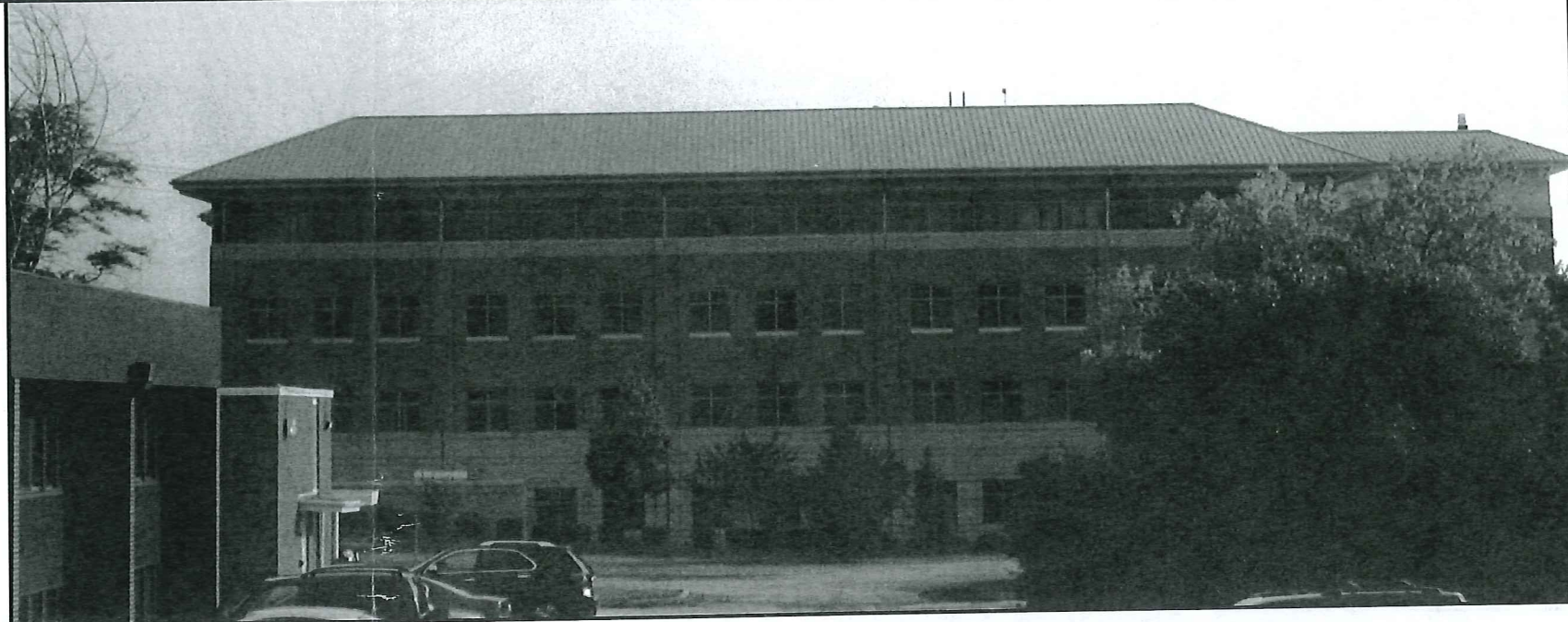
BUILDING ELEVATION (LOOKING NORTHEAST)
