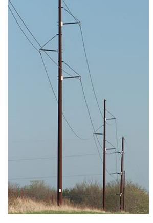
Some structures will have all the insulators on the same side of the structure in a vertical configuration
